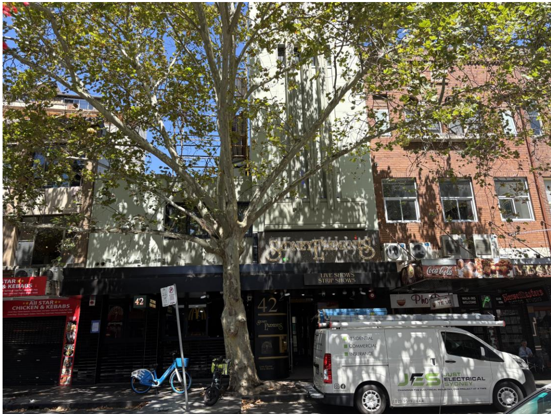
Figure 1: 42 Darlinghurst Road, Potts Point viewed from the north-west
